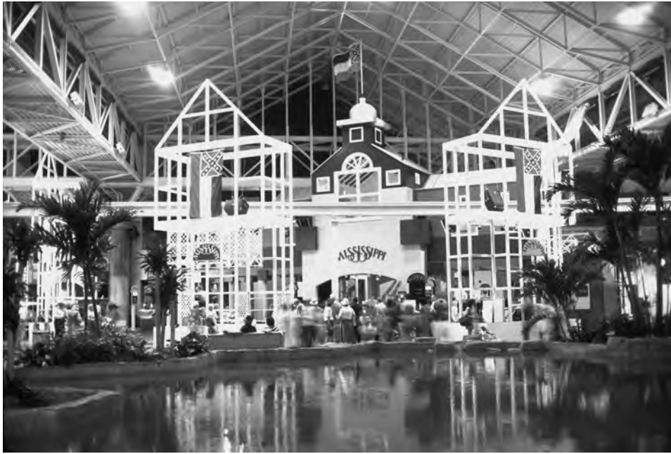
FIGURE 4. Mississippi Pavilion, New Orleans World Expo, 1984. Design by Mockbee Coker Howorth Architects, 3D International, and Communication Arts Company. Courtesy of Hap Owen of Communication Arts Company.
