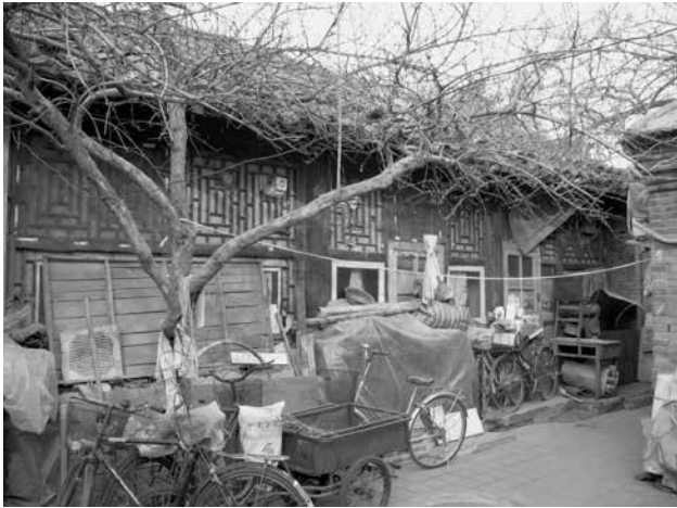
FIGURE 8. Dilapidated courtyard house on Qingfeng Hutong before renovation.
