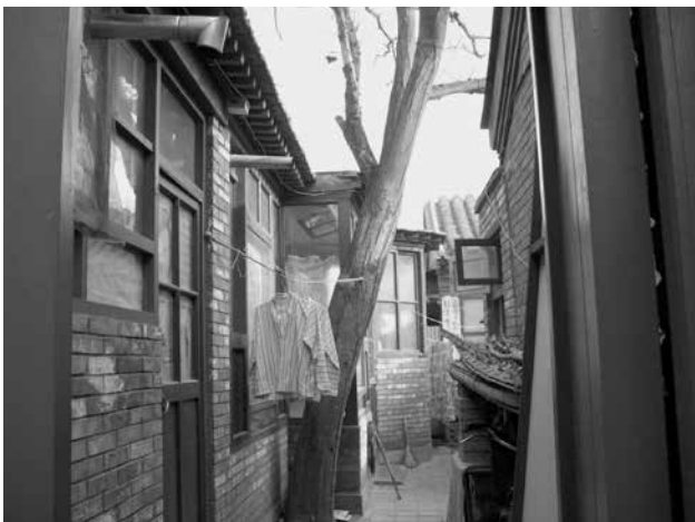
FIGURE 10. Renewed courtyard house on Suluobo Hutong with protruding building extensions that leave very little usable space.
