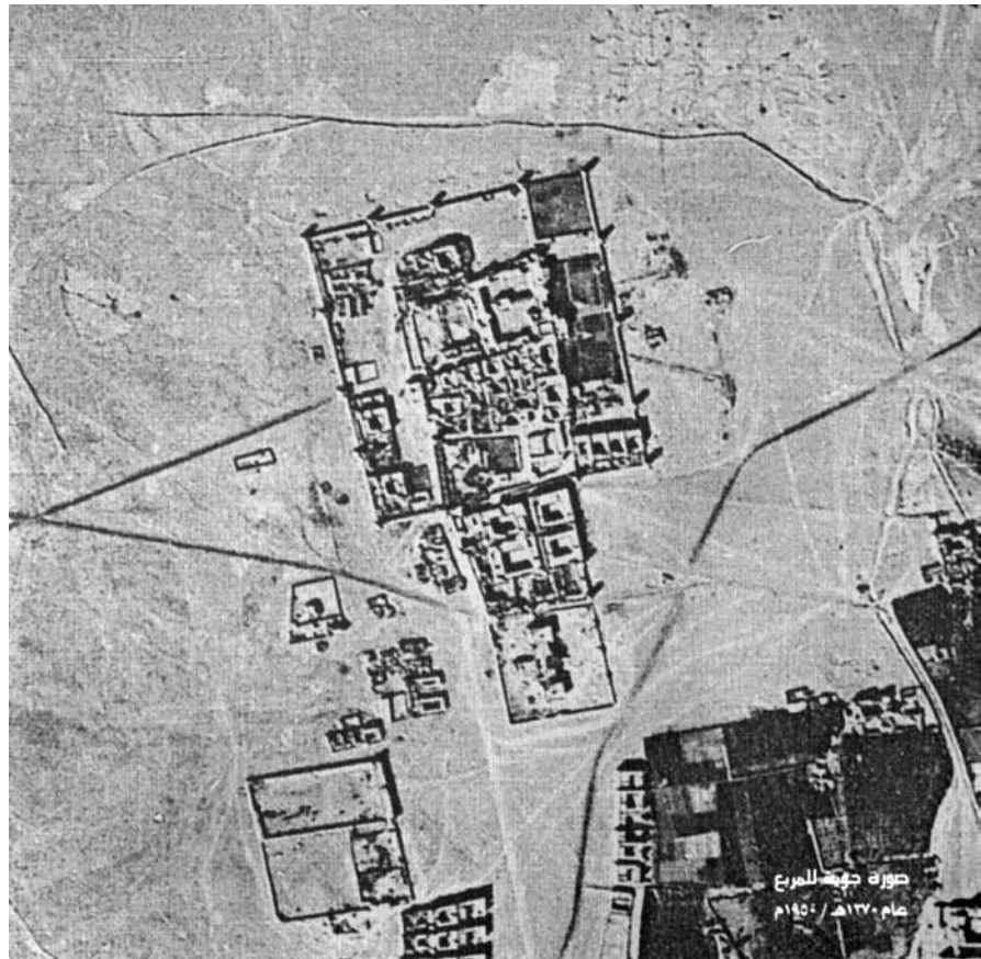
FIGURE 1. Aerial view of al-Murabba' Palace in 1950. Courtesy of Saudi Aramco.
