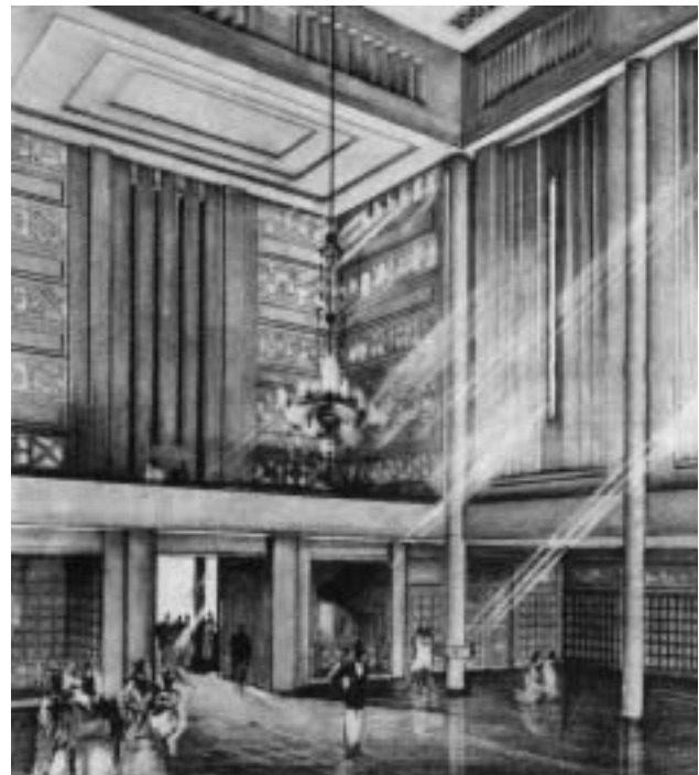
FIGURE 13. The entrance hall of the church at Morne à L'Eau. Thin columns emphasize the impressive elevation of the hall, while the thickness of the concrete walls disappears in the orchestration of pilasters and geometrical enrichments. This elaborate manner is extended to the ceiling, also carefully sculpted and hollowed. (Drawing by Ali Tur, in Encyclopédie de l'Architecture: Architecture Coloniale, Guadeloupe: Bâtiments gouvernementaux et communaux , Ali Tur, Paris, Editions Albert Morancé, 1930.)
