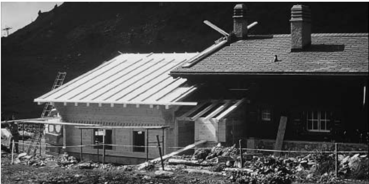
FIGURE 6. Building an extension to a chalet at the Col de Bretaye for rental during the tourist season. Vernacular building techniques are alive and in demand, in this case for the production of luxury chalets at a premium price. Constructor: Daniel Mermod.
