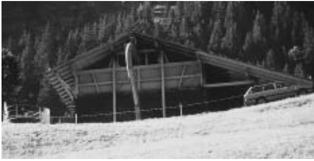
FIGURE 5. A new barn is built using frame construction, with the outer wall being “overclad” with logs. Gsteig.
