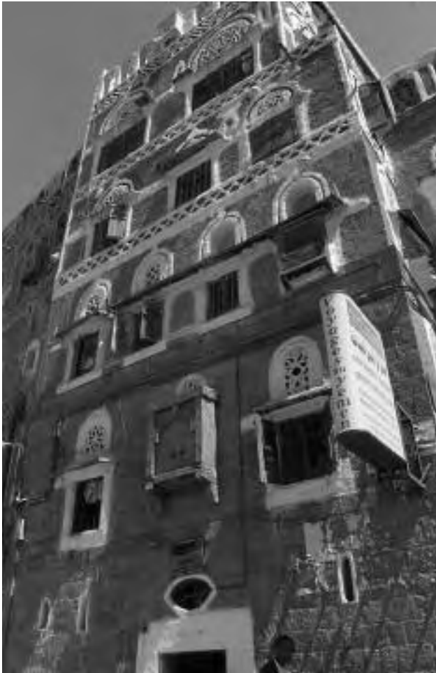
FIGURE 12. The upper floors of this house were built by the usta who served as consultant to the UNESCO Campaign.
