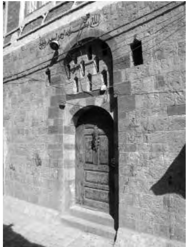
FIGURE 16 (RIGHT). A new door opening in a recent restoration, designed after the middle drawing in Figure 17 (the builder is the son of the usta whose work is shown in Figure 12).
