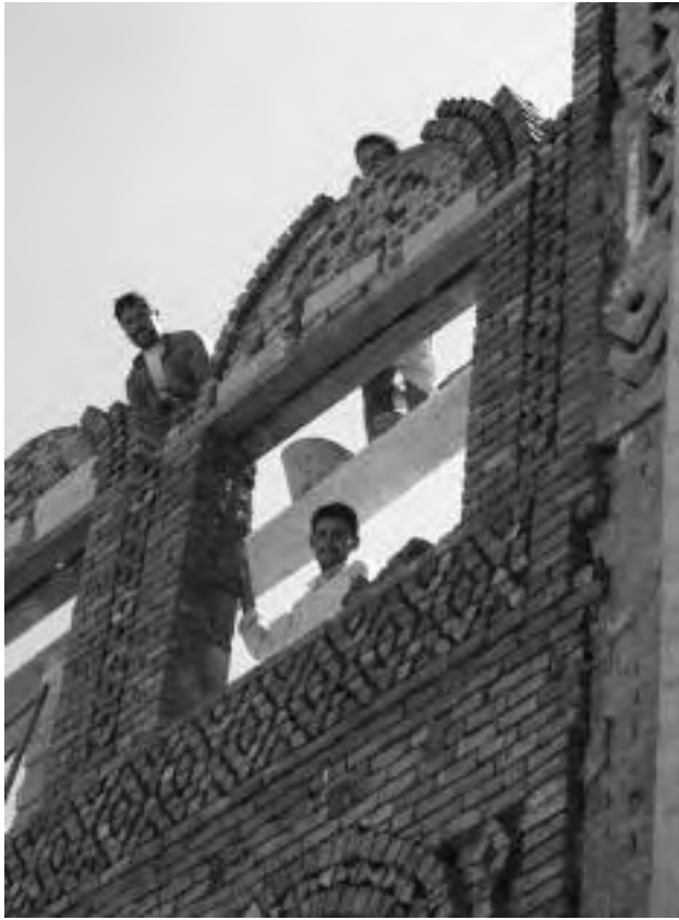
FIGURE 11. Brick arches and detailing applied as veneer on a concrete block wall.
