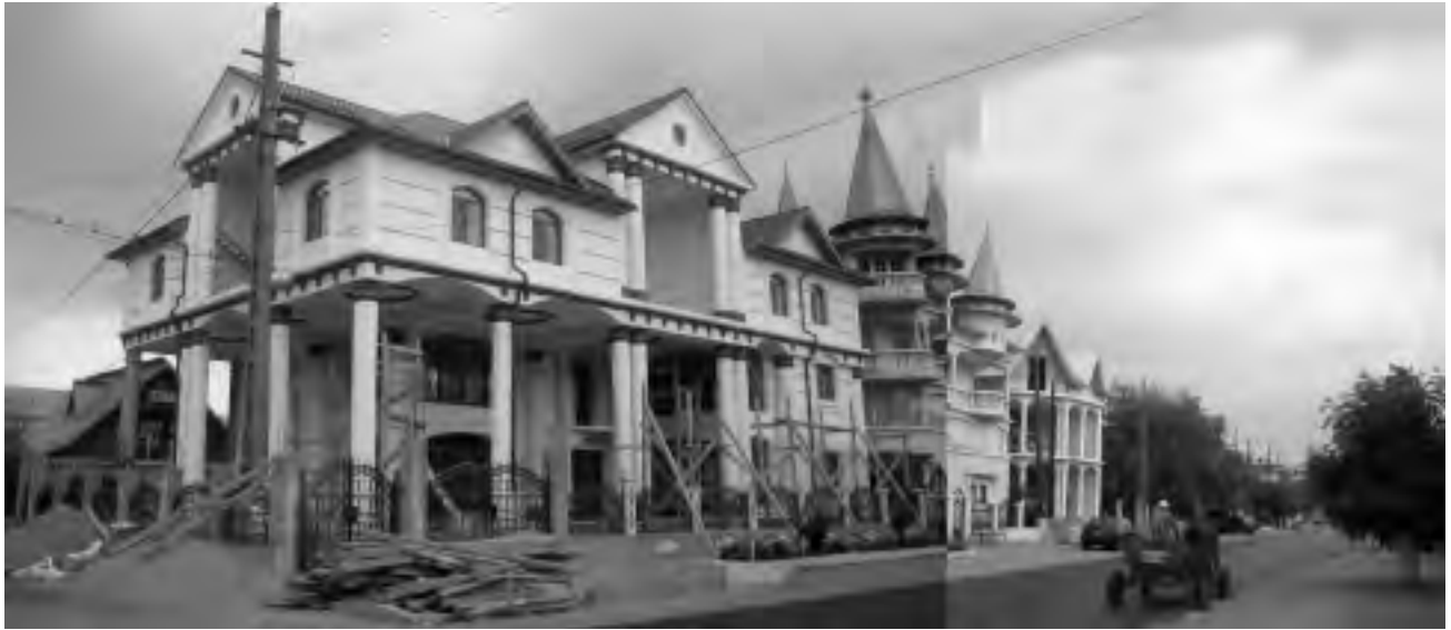
FIGURE 11. An example of a newly renovated palace with a colonnade in Buzescu.
