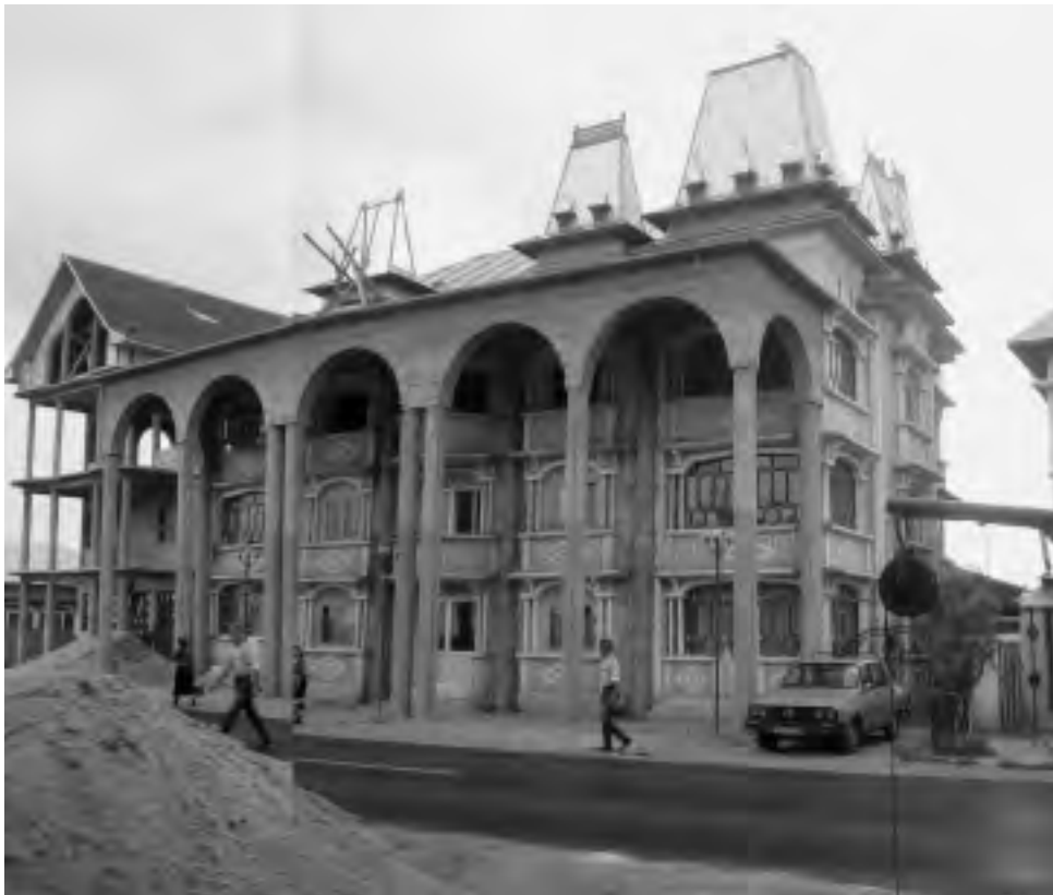
FIGURE 12. Residence under construction in Buzescu. The colonnade is applied on top of the old facade, blocking existing windows, leaving decorative dormers still visible in the back.
