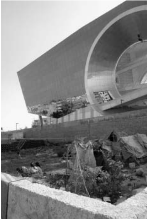
FIGURE 16. Infosys communications center with village land use in the foreground.
