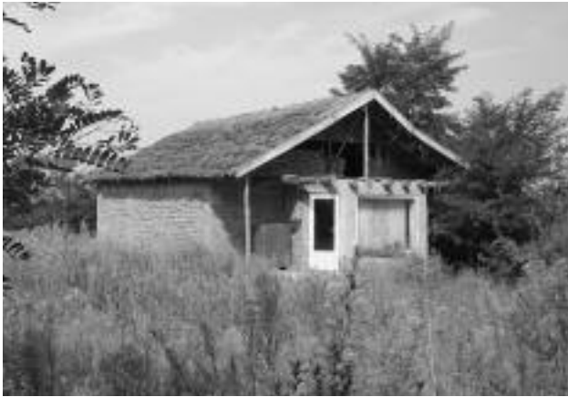
FIGURE 15. A new, unfinished house using adobe and thatch, but also thermal-insulating double-pane windows and doors. Topalu, Constanta, 2005
