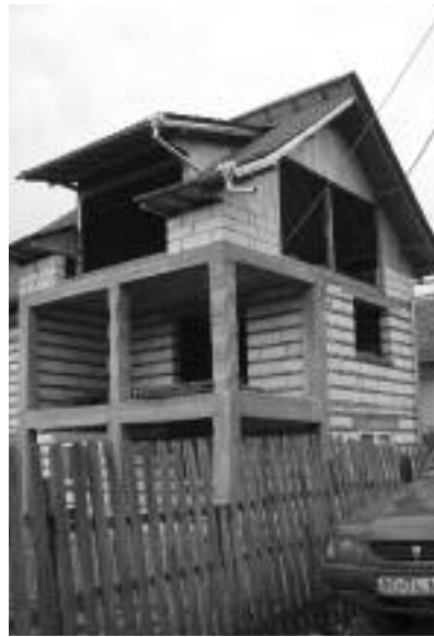
FIGURE 10. Alternate layers of red brick and white cement blocks used in a new house, Corbsori village, Arges, 2007.
