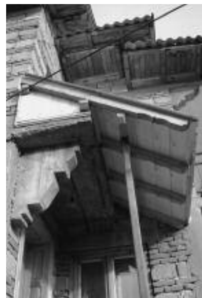
FIGURE 11 (ABOVE). The use of concrete to resemble the typical details of a timber structure, Corbsori village, Arges, 2007.
