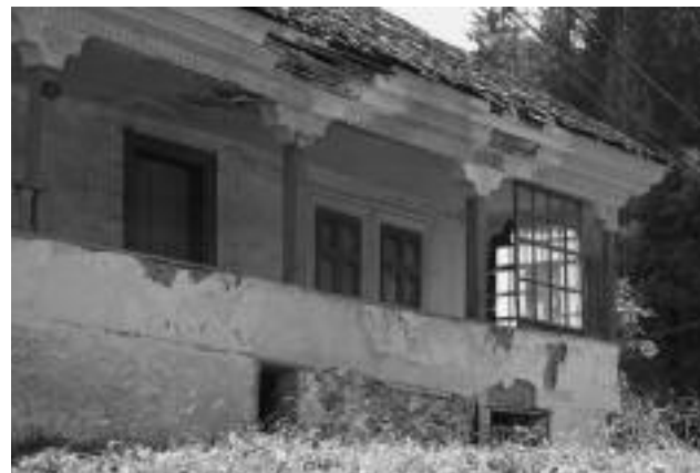
FIGURE 5. Abandoned house in Dambovicioara, Prahova, 2007.
