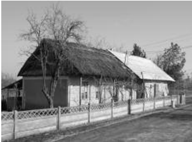
FIGURE 3. The use of reed thatch vs. corrugated metal sheets as a roofing material in the village of Murighiol, Tulcea, 2006.
